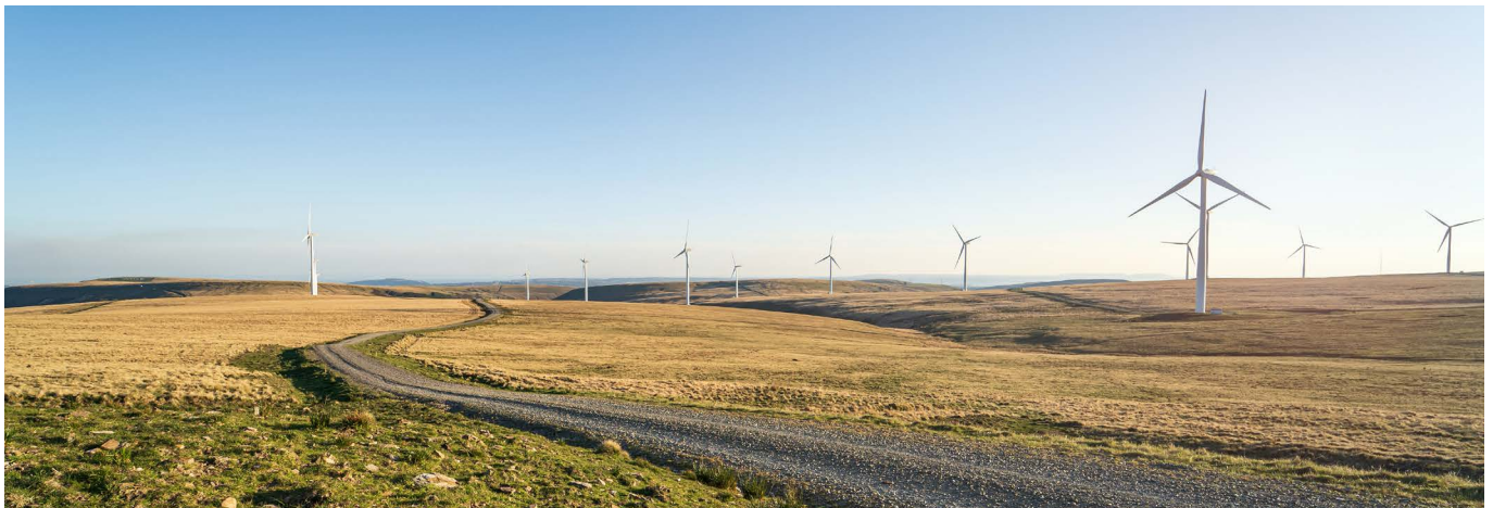
Mynydd y Betws Wind Farm, Swansea
